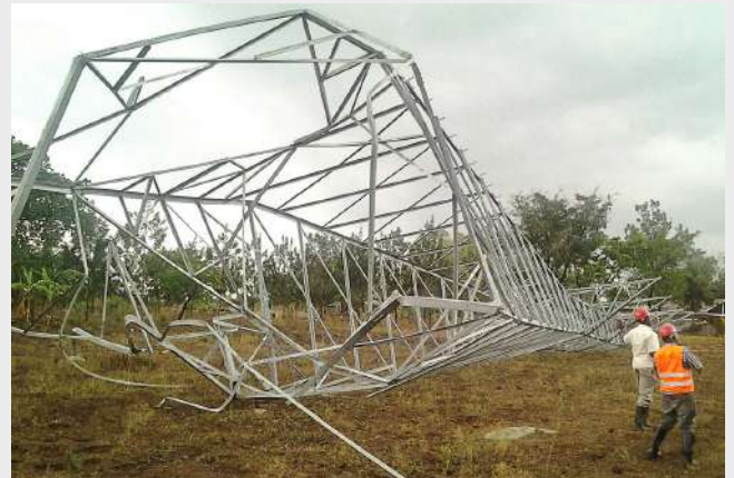
Collapse of a 132kV tower after bolts and crossmembers were removed to sell as scrap.
